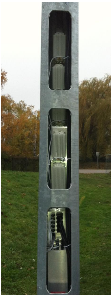
Attached mast boxes with operating devices
