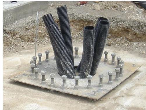
Foundations with anchor basket
